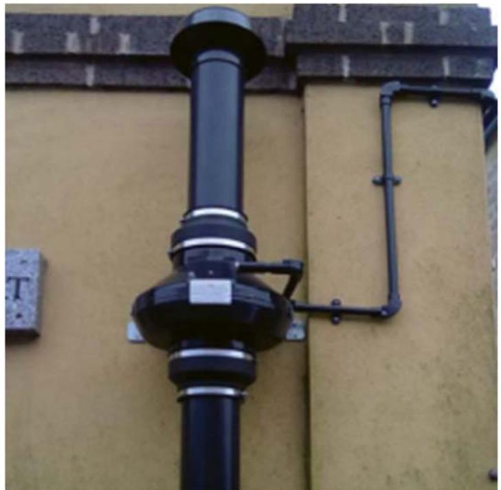
**IMPORTANT:** After installation, the fan wiring enclosure should be sealed with silicone sealant to ensure water cannot get in and damage the fan.
